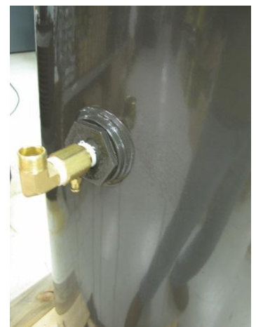
Discharge air line removed from check valve.
