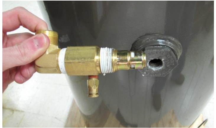
Existing check valve removed from tank.
