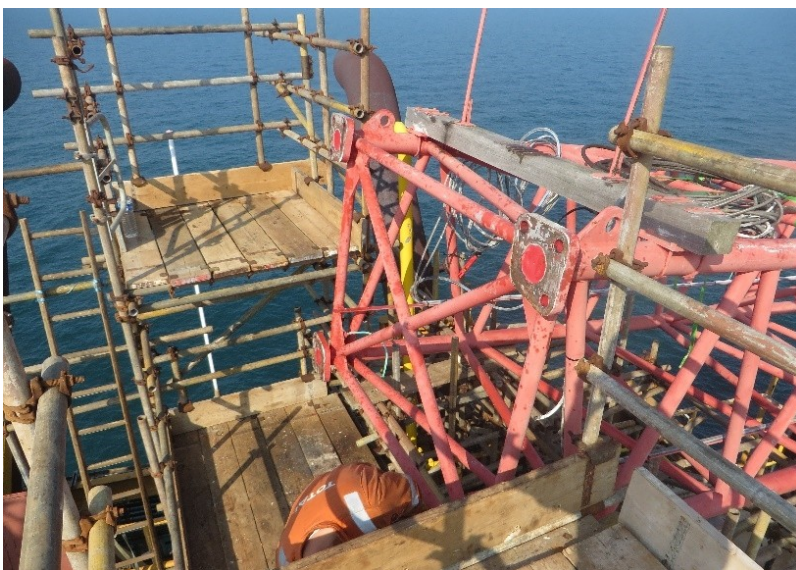
Photo: Deck crane without crane boom tip
