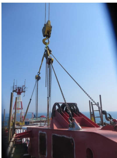
Photo: Lifting configuration attached to the old crane boom tip
