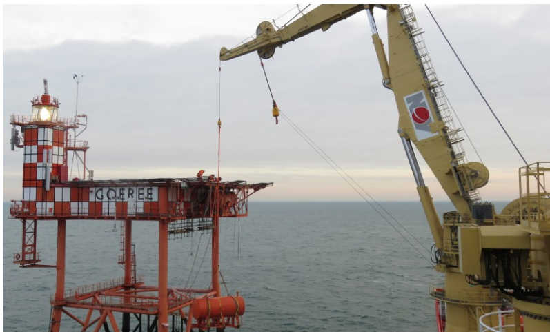
Picture: offshore lifting of diesel tank
