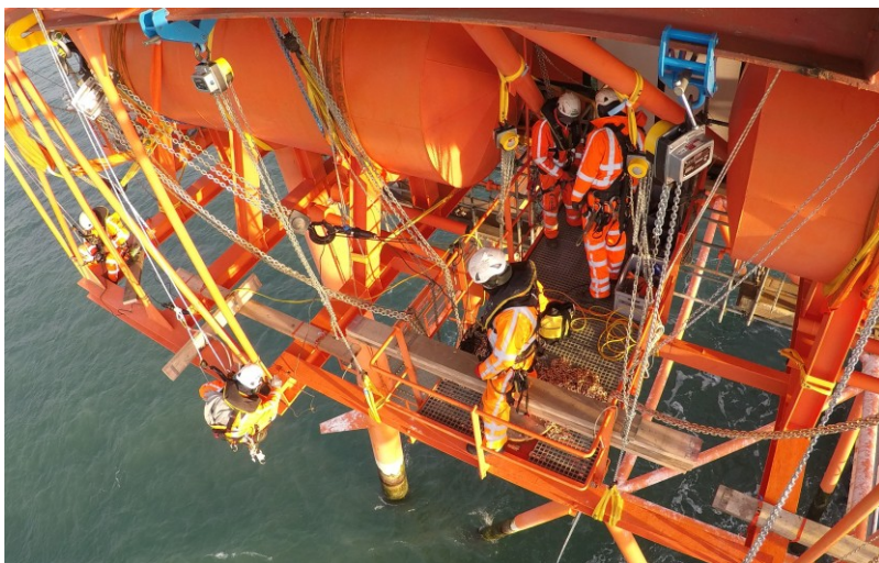
Picture: Preparing rigging and cutting steel
