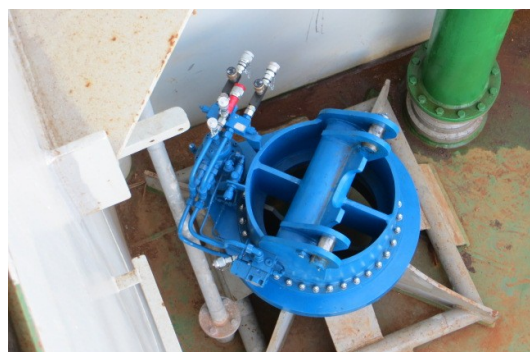
Pictures: Equipment preparation and installation
