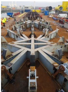
Picture: Barge with type 2 grillage
