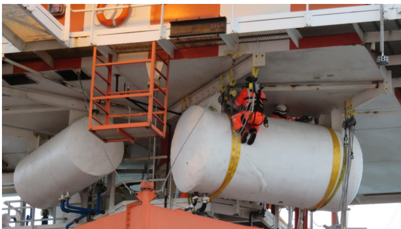
Picture: Preparing rigging old diesel tank
