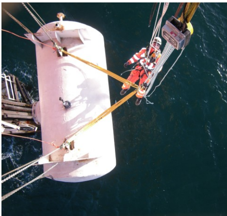
Photos: Rigging and offshore lifting of the diesel tank
