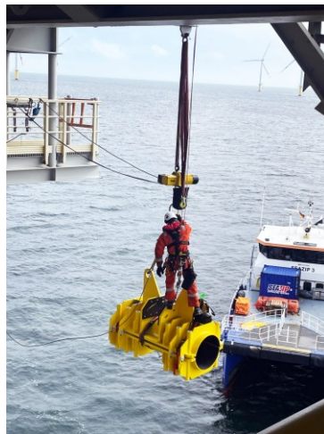
Rope access during cross hauling
