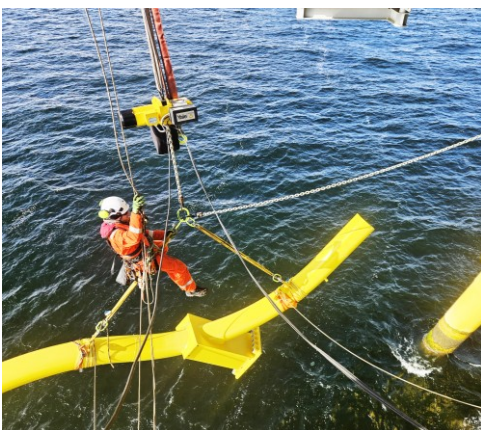
Rope access during cross hauling
