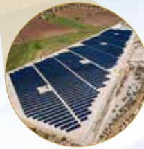
Kahramanmaraş DOKUBOY ARAZI GES 17.000 kWe / 20.999,94 kWp
