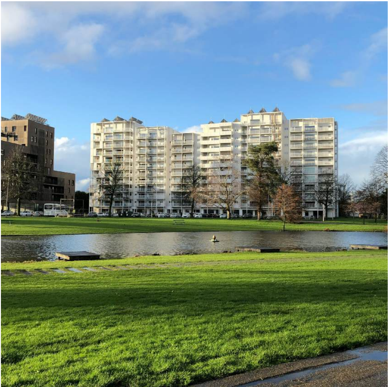
Drie Hofsteden retrofitting in Kortrijk, Belgium © Agata Smok
