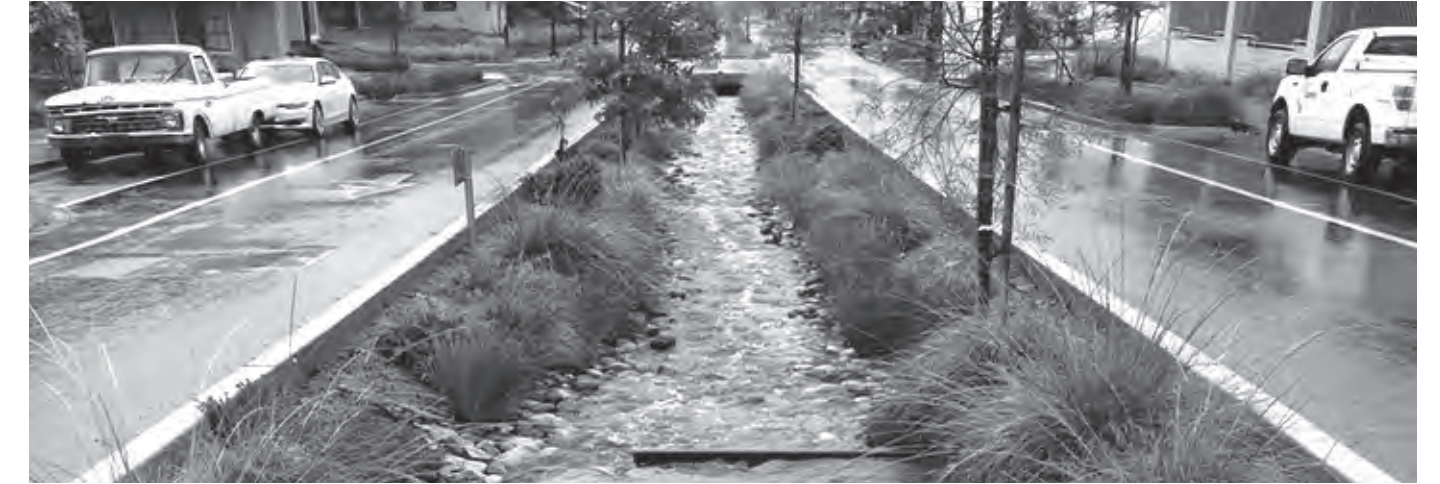
Bioswales on 21 st Street, Paso Robles, CA (Image Source: SvR Design Company)
