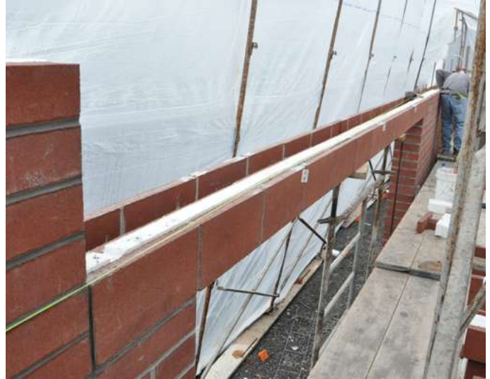
HI-R/HI-R-H Closed Bottom Lintel – Pre-fabricated installation
