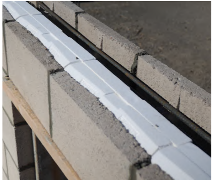
HI-R-H units reinforced as a lintel before placement of succeeding courses
