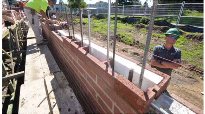
Jambs being constructed using HI-R-H Half High Sash/Jamb Unit
