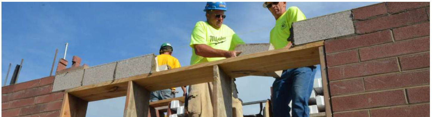
Traditional masonry lintel installation using a form (this lintel is not insulated)
