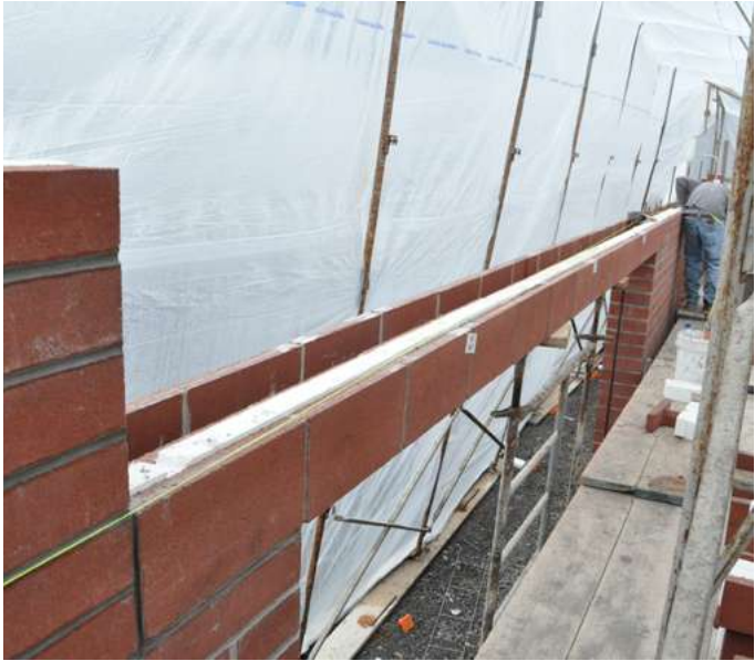
HI-R/ HI-R-H Closed Bottom Lintel – Pre-fabricated installation
