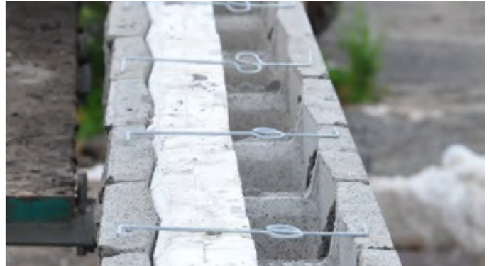
HI-R-H Units with Rebar Positioners – Prior to Grout
