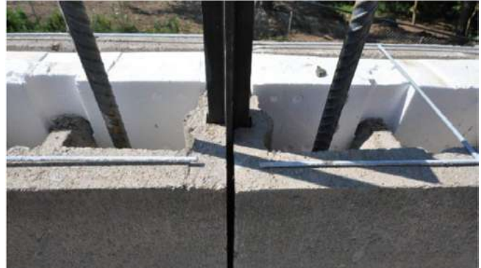
Control joint using HI-R-H Sash/Jamb Unit
