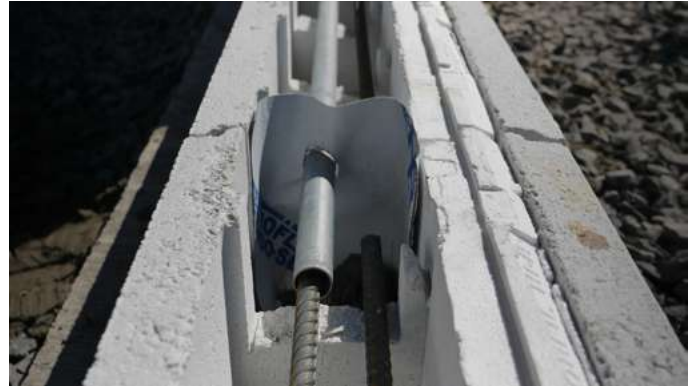
Bond break at Control Joint
