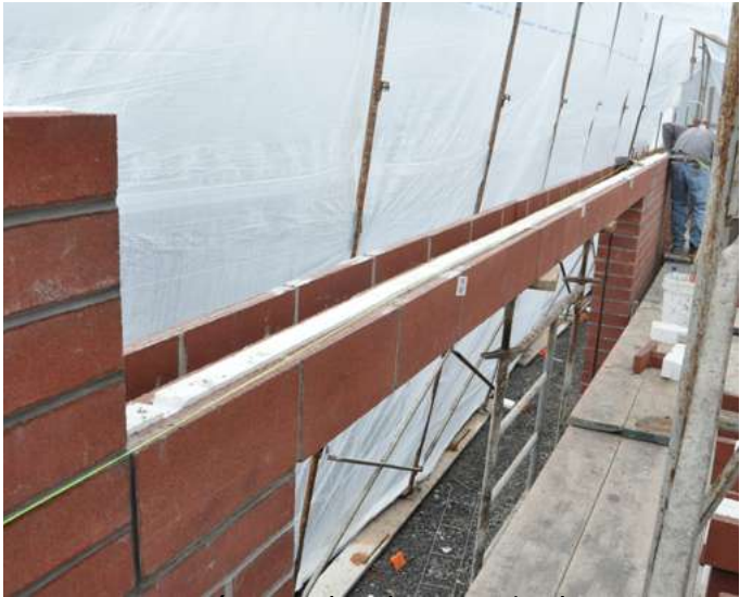
HI-R/HI-R-H Closed Bottom Lintel – Pre-fabricated installation
