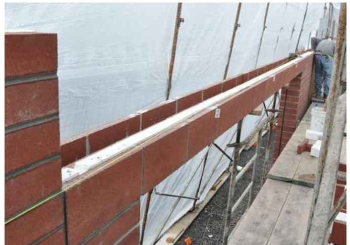
HI-R/HI-R-H Closed Bottom Lintel Pre-fabricated installation
