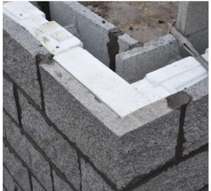
Corner with L-shaped fitting cut from CMU and soap. The HI-R-H unit to right's face shell can be cut as needed. This detail can be used with both HI-R and HI-R-H units
