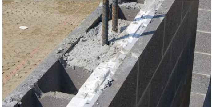
Partially Grouted HI-R Wall
