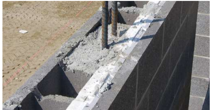
Partially Grouted HI-R Wall (shown with 12×8×16 unit)
