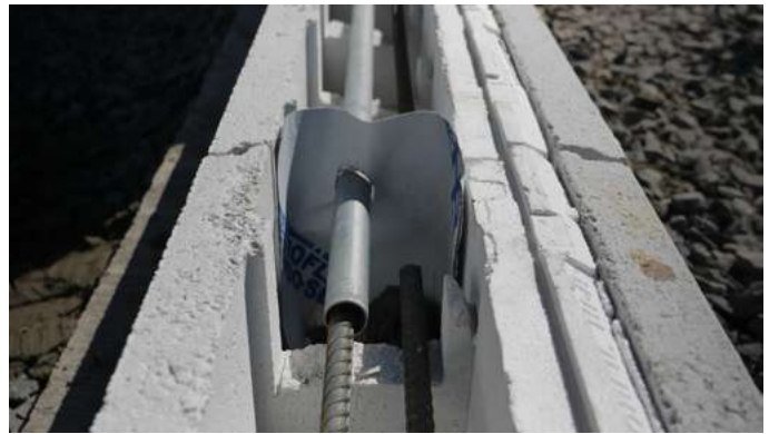
Bond break at control joint
