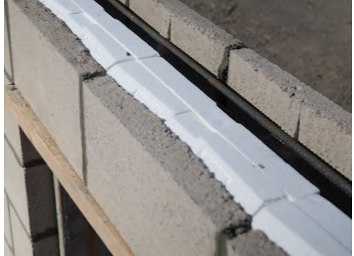
HI-R-H Unit reinforced as a lintel shown prior to grouting
