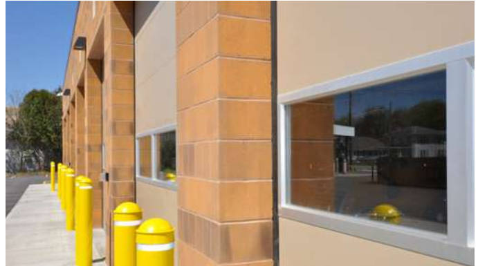
Finished Door Jamb using HI-R-H Sash/Jamb Unit
