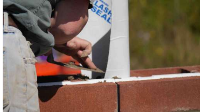
Bond break at control joint
