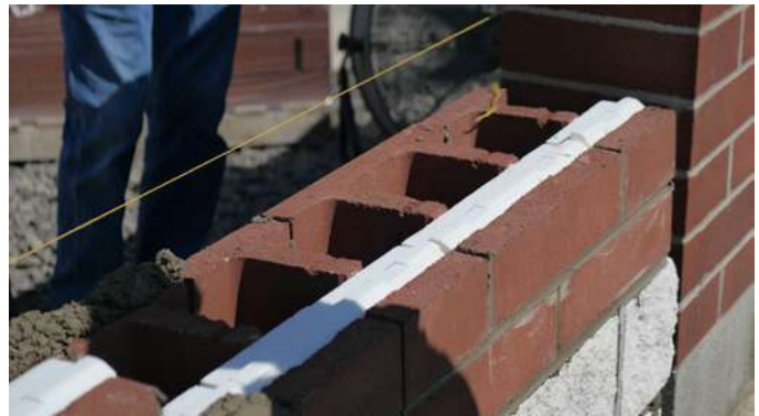
HI-R Half High Wall Under Construction
