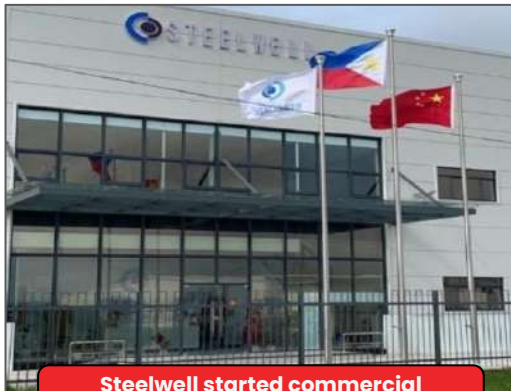
Steelwell started commercial operations in LIMA Estate on Jan'25
