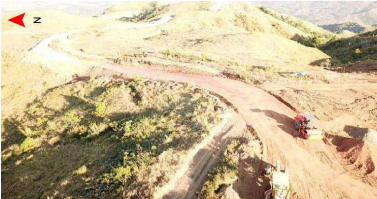
Road grading at PV plant site
