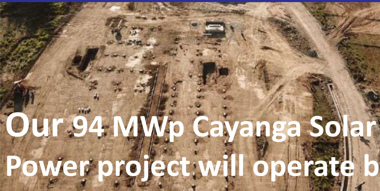
Establishment of foundations for temporary office
