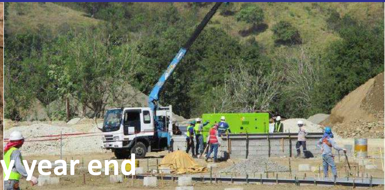
Temporary office pedestal installation
