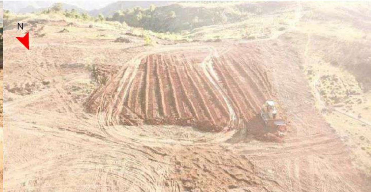
Grading works at the substation area
