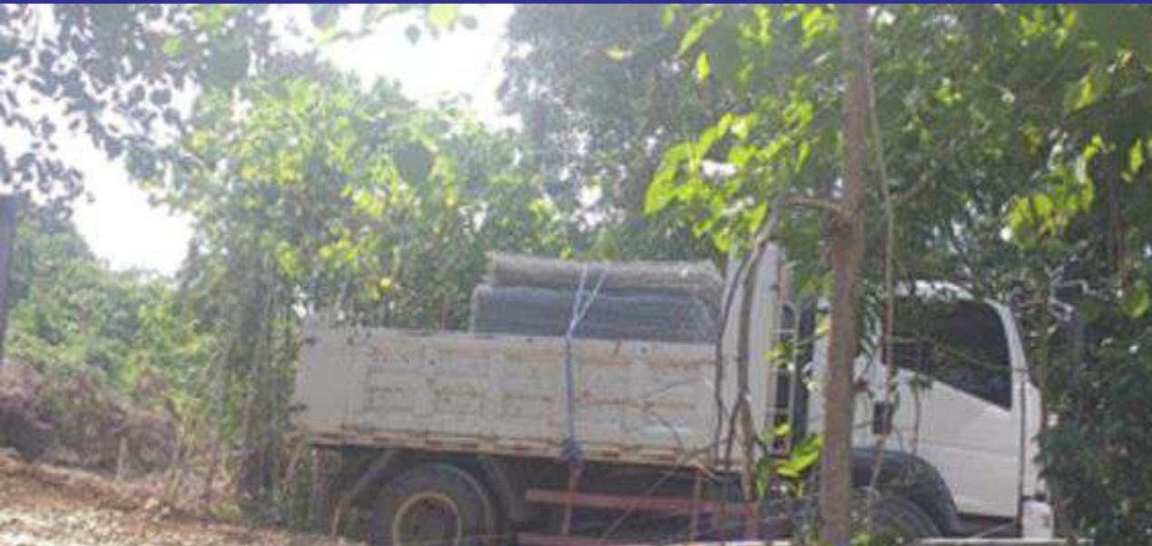
Delivery of slope protection materials
