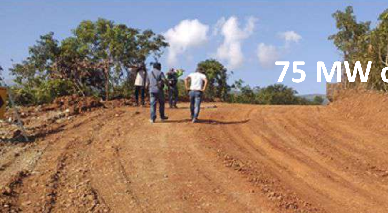
Joint inspection of excavation limits
