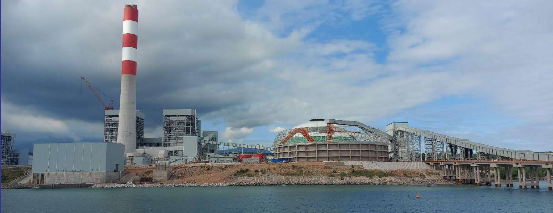
Plant View From Jetty
