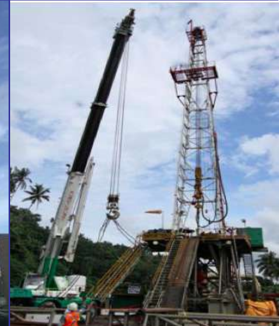
Tiwi Make-UP Well Drilling Rig in Operation
