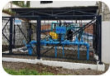
Installation of new wells and transmission mains
