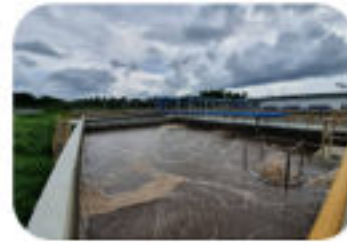
Upgrade of Sewage Treatment Plant
