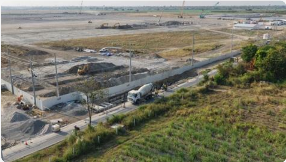
Accelerated development of spine road connecting expansion area further sustaining momentum
