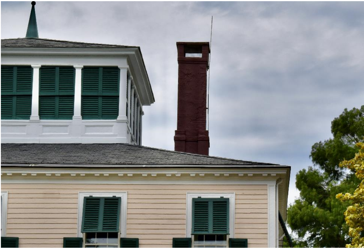
Fig. 20. North Elevation - note location of built-in gutter where the slate stops at the eave
