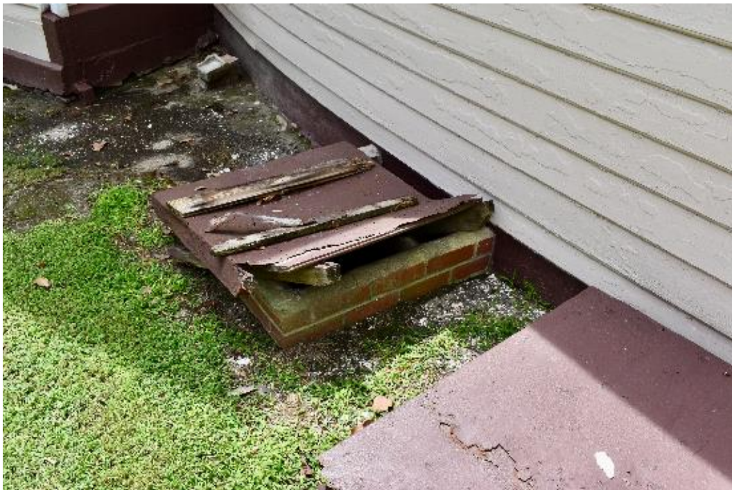
Fig. 26. Covered foundation vent - north elevation of hyphen
