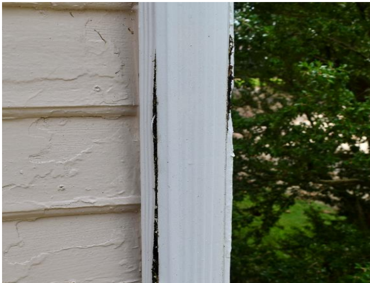
Fig. 21. Clogged downspout – note split in downspout.
