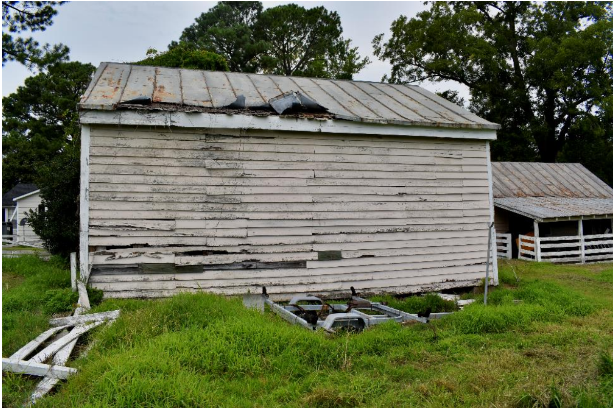
Fig. 31. East Elevation Carriage House/Barn
