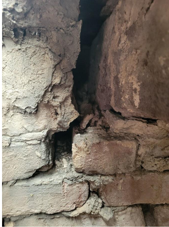
Figure 15 South Stairs Stone Step and Header
