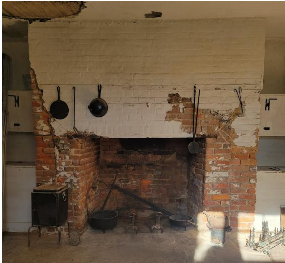
Figure 3 South Room Facing Chimney Block
