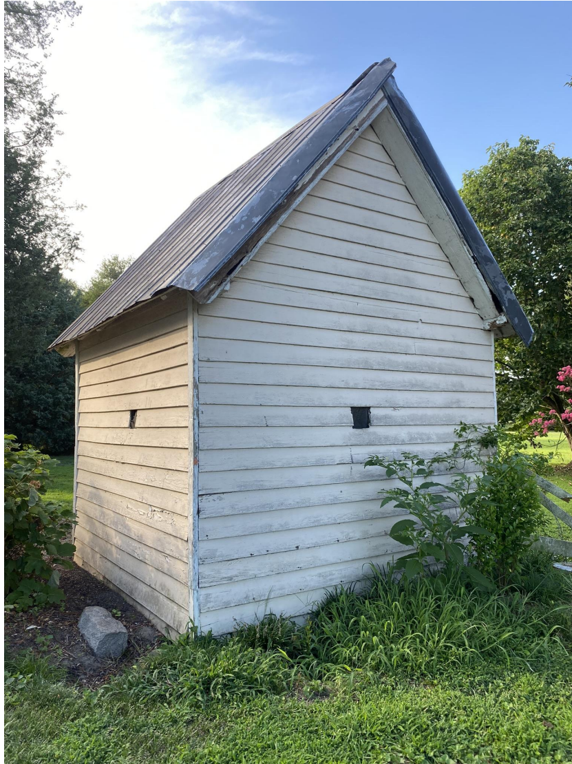
Hayes Smokehouse rear. Note holes cut in siding.
