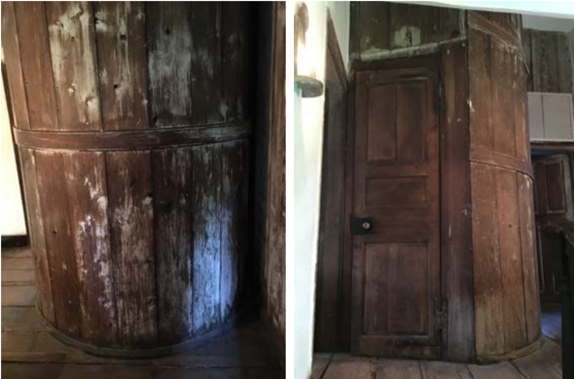
Third-floor Surround for Attic Stair
