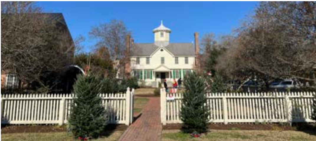
The Cupola House December 2024 Site Visit
