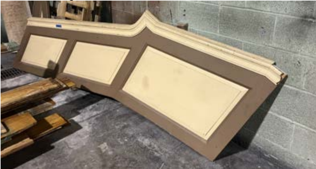
Wainscot with original section of chair rail
