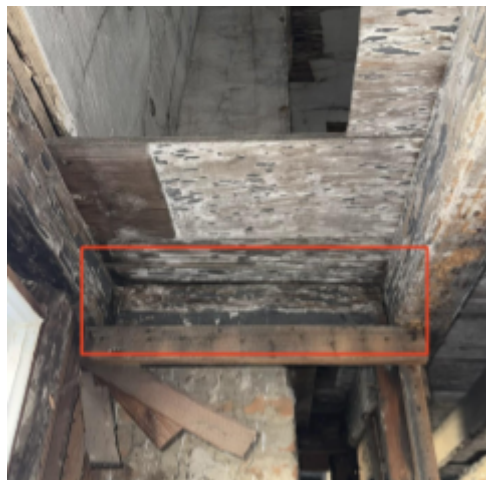
Fig. 53. Possibly original second floor hearth trimmer notched to header and joist.
