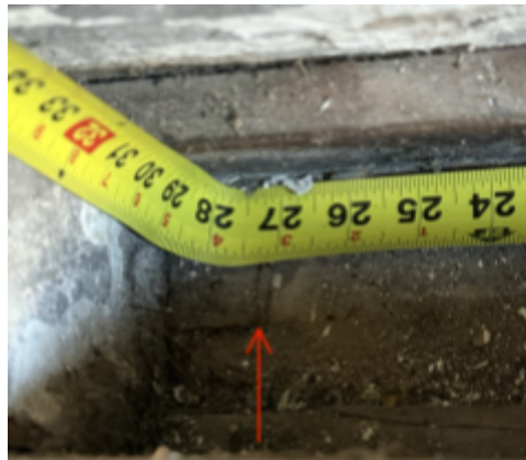
Fig. 14. Original post location with 27" spacing.
