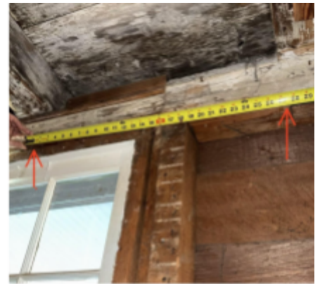
Fig. 15. Mortises with 27" spacing on west side of north wall.
