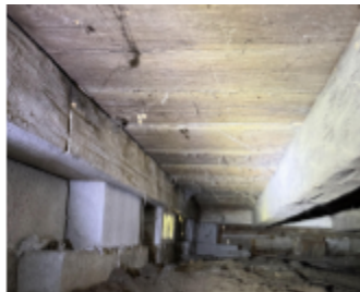
Fig. 3. C1719 west sill and joist with no notches to accommodate a chimney or hearth.
