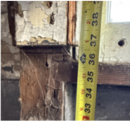
Fig. 13. Sill notch in identified c1719 post.
