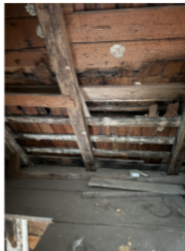
Fig. 38. Core rafters with Later shingles and lath spaced 8" under porch roof.
