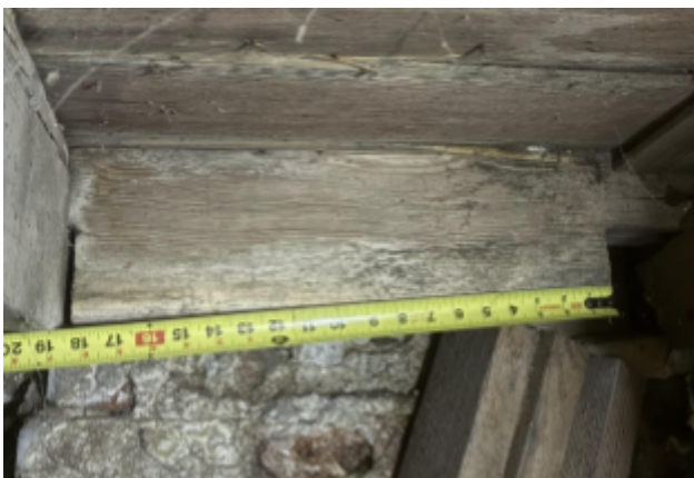
Fig. 46. Hearth trimmer on east wall.
