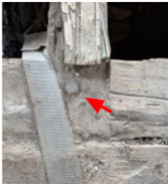
Fig. 2. Pinned lap joint of c1719 floor joists.
