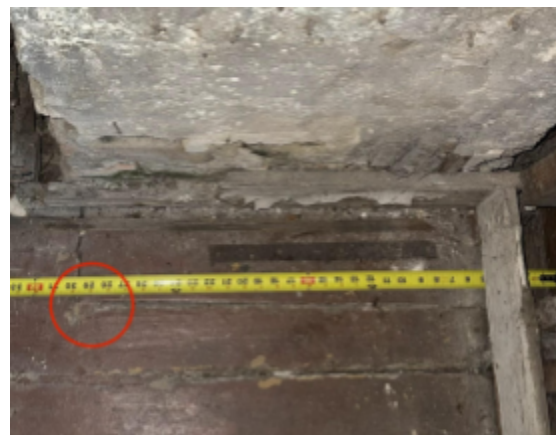
Fig. 47. Early hearth evidence seen in replaced flooring, note miter circled in red.
