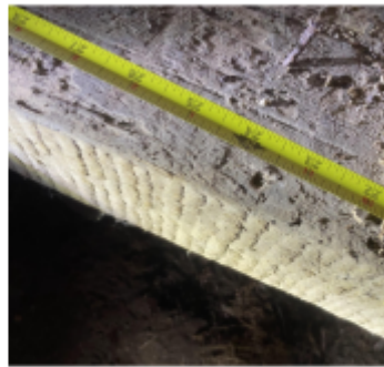
Fig. 8. Shed sill with straight sash saw marks.
