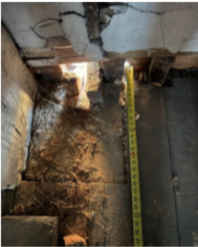
Fig. 51. Loft hearth evidence found in flooring.
