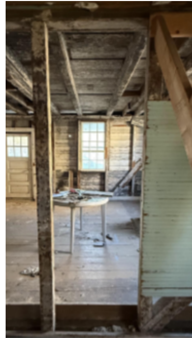
Fig. 23. South wall studs spaced 27" mirroring north window, east of door.
