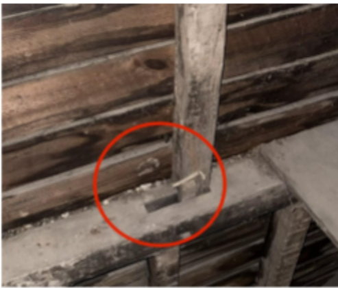
Fig. 48. Northwest mortise in header shown with gable post in situ.
