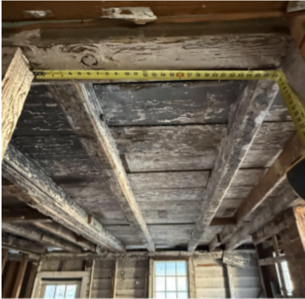
Fig. 22. South studs with 27" spacing mirroring north window location east of door
