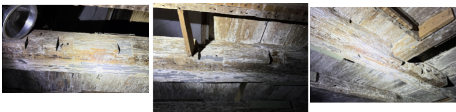
Fig. 41-43. North, center, and south sections of header with lap joint notches for early partition wall. Note presence of early lime wash inside notches.
