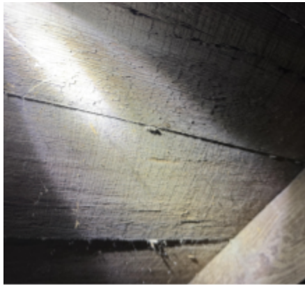
Fig. 10. Bottom side of early, possibly original, pit sawn flooring on west side of core.
