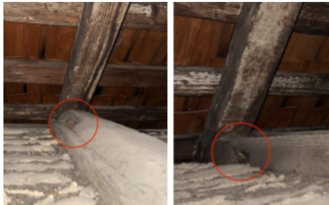
Fig. 44-45. Beveled lap notches in collar ties for loft partitions east and west of access well.
