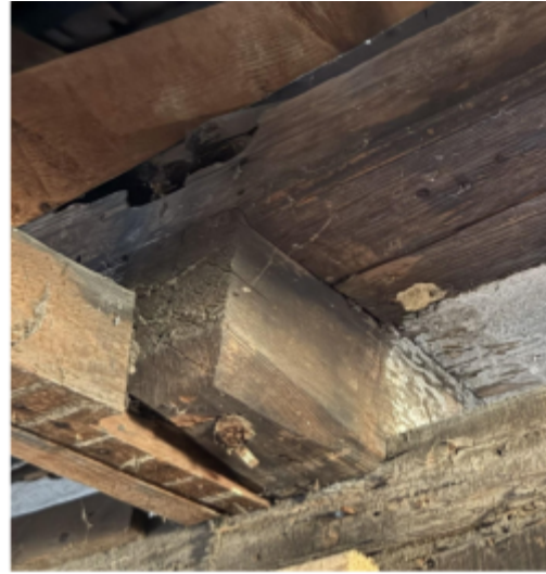
Fig. 37. c1719 south cornice with rafter notched to the thick molded edge pinned false plate.
