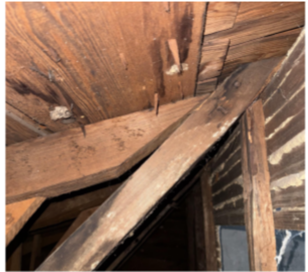
Fig. 33. 19th c. sash sawn shed rafter nailed to the top of c1719 rear rafter.
