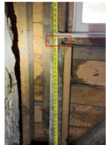
Fig. 18. Notch in post with corresponding mortise in east gable header to south of fireplace indicating an early window opening.
