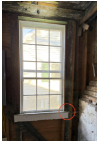
Fig. 17. Notch in post mortised to east gable header to north of fireplace indicating an early window opening.
