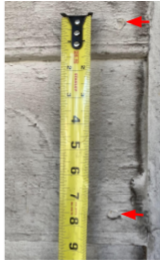
Fig. 28. Northeast siding with wrought nails at @. 8" vertical spacing.
