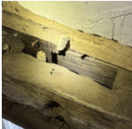
Fig. 49. Northeast large mortise in header with gable stud in situ.
