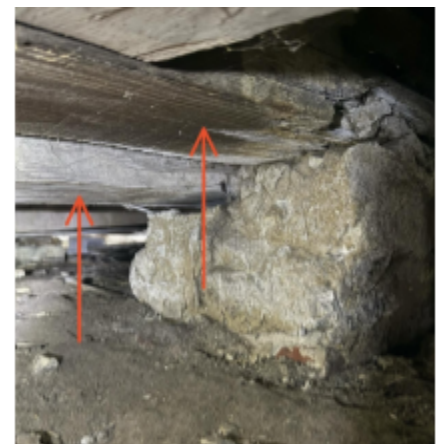
Fig.1. Bermuda stone and brick pier supporting sills for the c1719 core rear sill (r) and 19th c. shed front sill (l).
