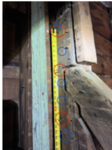
Fig. 27. Southwest corner post south face with siding nails at @ 8" vertical spacing (red) and earlier(?) smaller nails spaced approximately 5" (blue).
