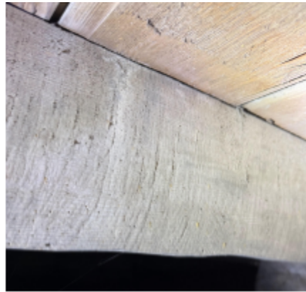
Fig. 11. c1719 pit sawn joist with later sash sawn gauged flooring on east side of core.
