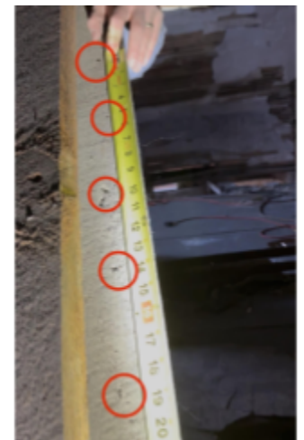
Fig. 39. Top side of core south rafter with 5" nail spacing from original roofing material.
