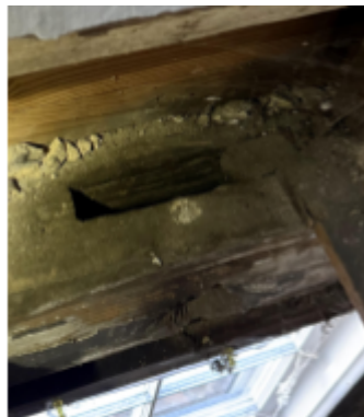
Fig. 25. Large southeast mortise with a possible cut off tenon still inserted.
