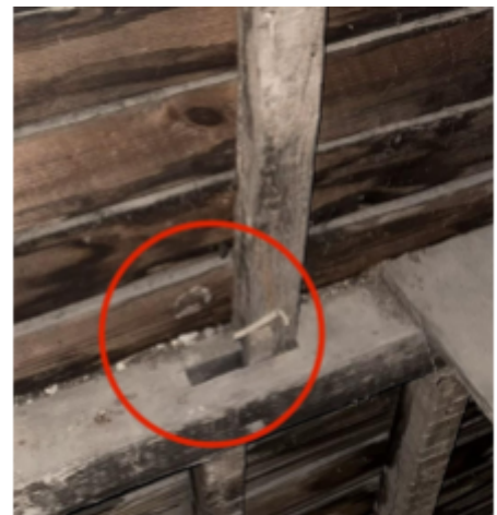
Fig. 26. Northwest large mortise with gable stud from top.
