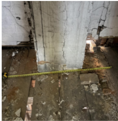
Fig. 51. Loft hearth evidence found in flooring.
