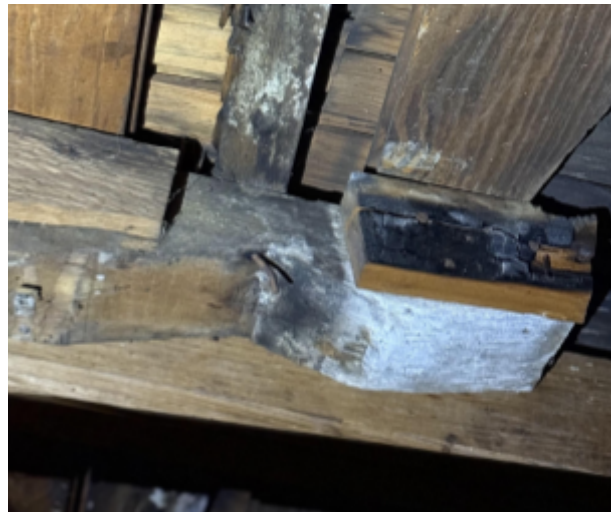
Fig. 35. 19th c. shed rafter tails that once extended over their header. Note original cut nail.
