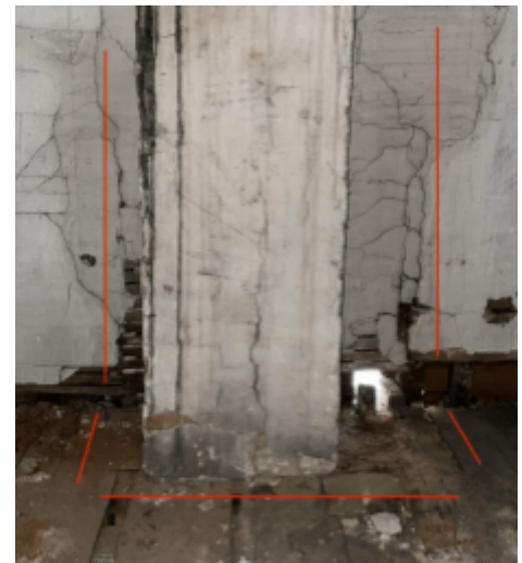
Fig. 52. Loft fireplace location outlined in red.
