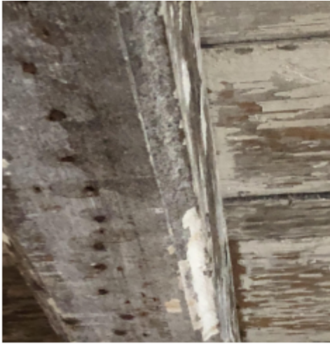
Fig. 36. Ogee molded edge of joists.
