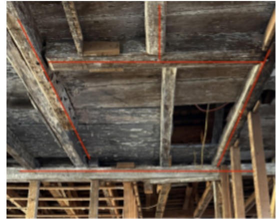
Fig. 40. Loft stair/ladder well. Original material marked in red.
