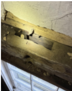
Fig. 24. Large northeast mortise with gable stud tenon inserted.
