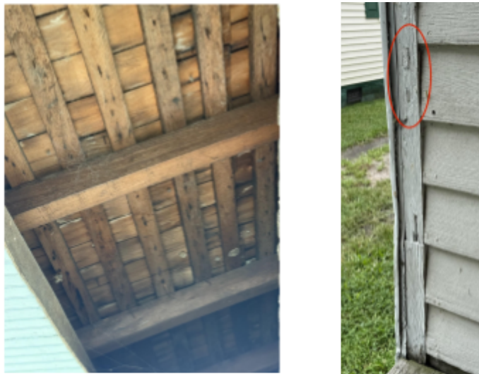
Fig. 54-55. Porch rafters in sash sawn cypress and cut off rail tenon on left post.
