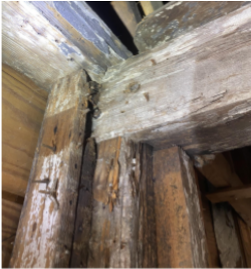
Fig. 29. Southeast post with later nailer for sheathing.
