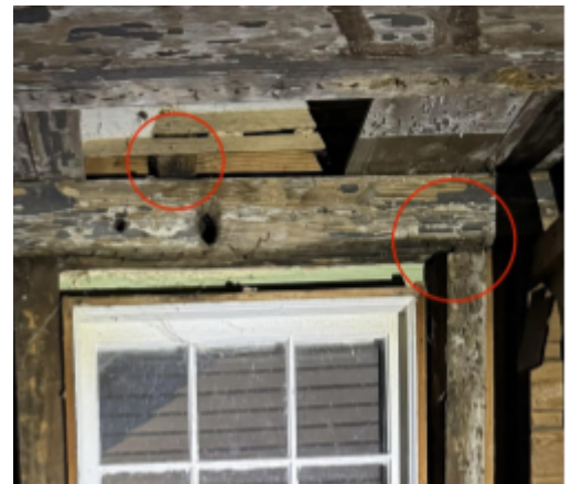
Fig. 50. In situ posts mortised into north end of east header.
