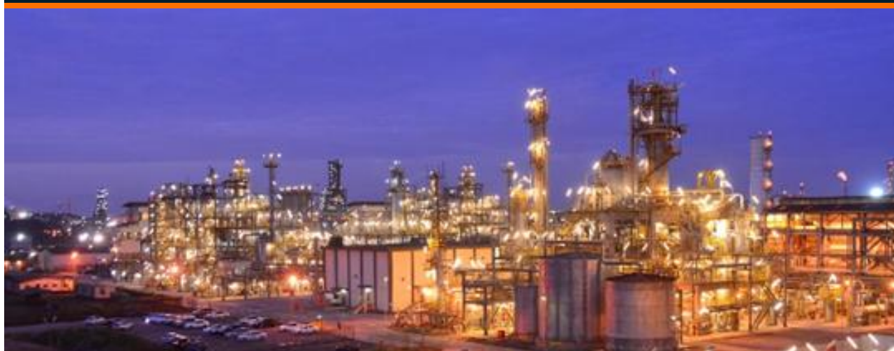
Trinidad production facility.
