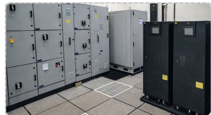
BPE Modular UPS Installation
