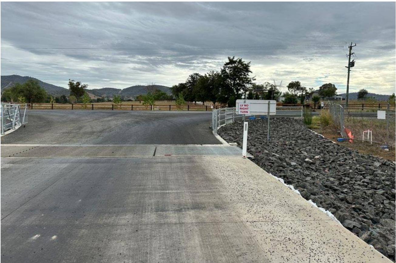
Photo B10(c)(viii)-1: Mud tracking minimal on Calala Lane
