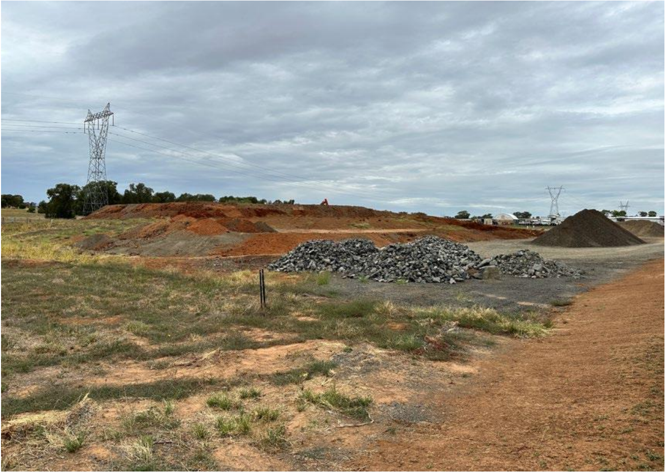
Photo B11-4: Topsoil and aggregate segregated from excavated materials
