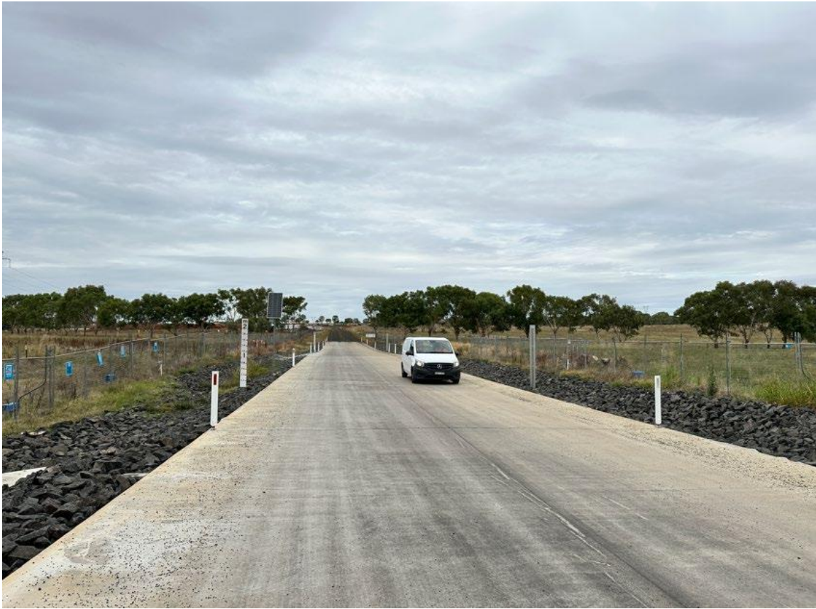
Photo B28-1: Stormwater controls observed onsite
