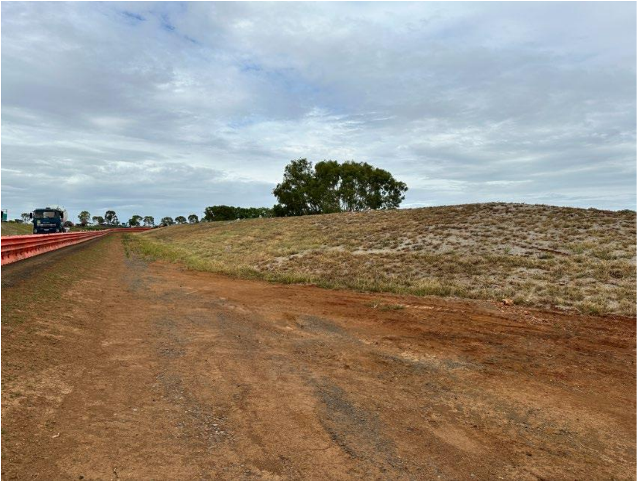
Photo B12-1: Embankment stabilised with sterile grass
