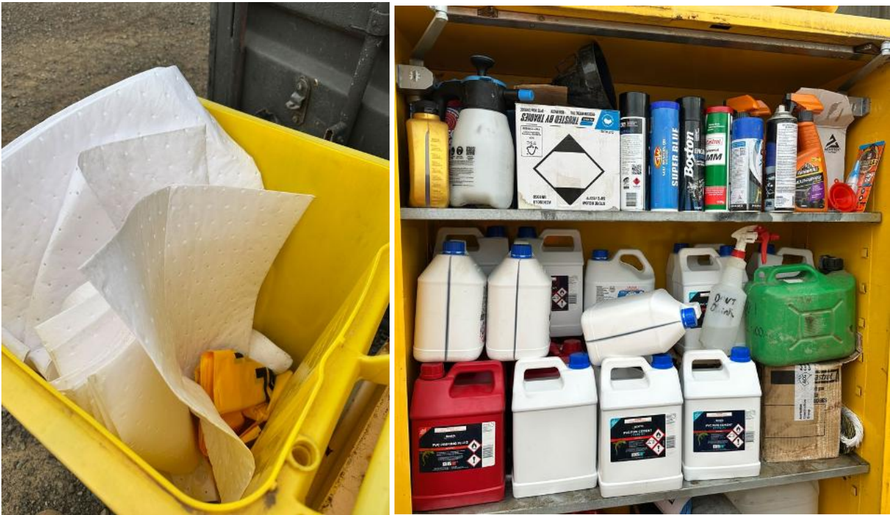
Photo B31-1: Chemical storage cabinet; drip tray; and provision of spill kits
