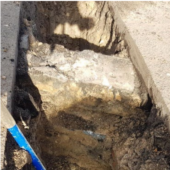
Photo 14 Wall footings (stone/sandstone)
