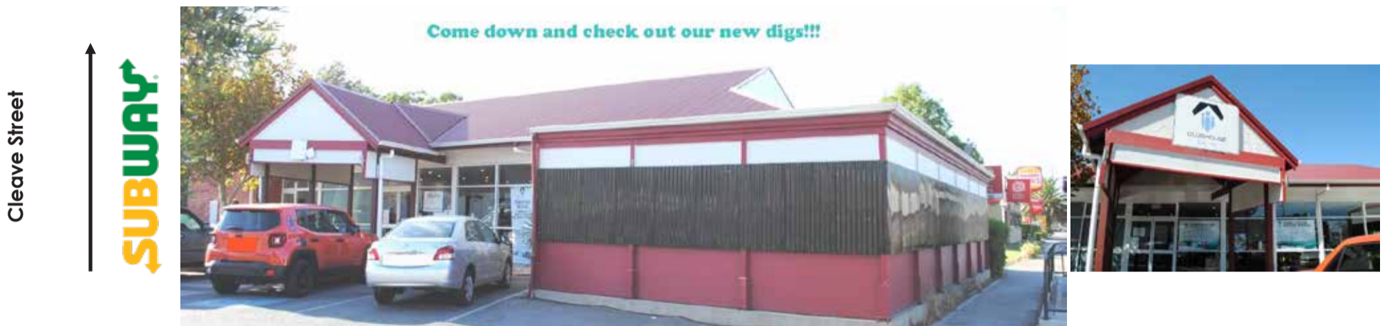
2 Cleave St Port Adelaide. ( behind Subway)
