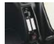
Central fuse box located behind seat
