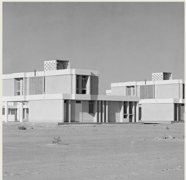
Photo of Prefab Housing Project (1970), Abu Dhabi. Source: AGDA Arabian Gulf Digital Archives
