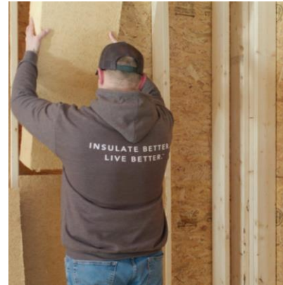
TimberBatt Wood Fiber Batt Insulation Install (Photo from TimberHP)
