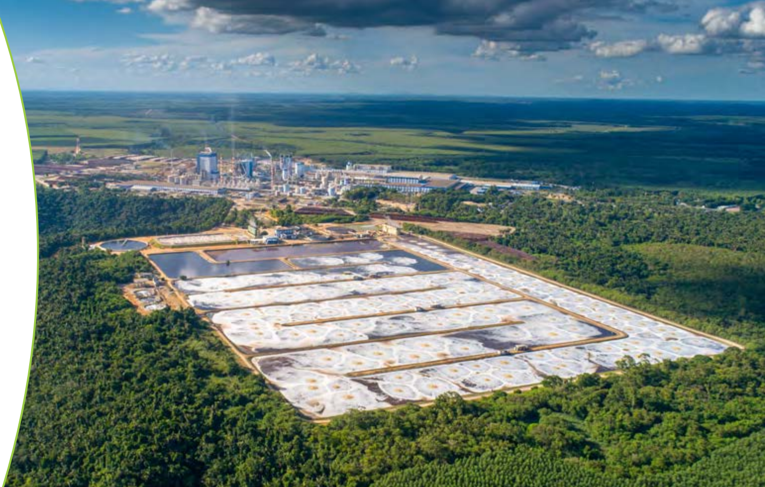
Effluent Treatment Area, Mucuri Unit (Bahia state). Photo: Ricardo Teles
