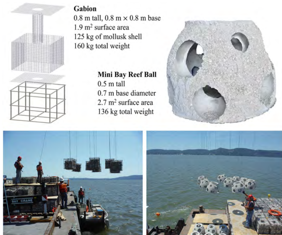
Figure 3. Top: shell-filled gabions and Mini-Bay Reef Balls used in full-scale construction. Bottom: deployment of the two substrate types, gabions and Mini-Bay style Reef Balls in July 2018 (photos by Brian DeGasperi/NYSDEC).
