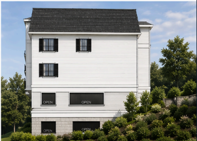
NORTHEAST SIDE VIEW
