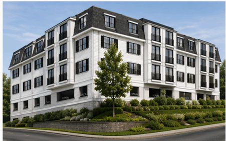
SOUTHEAST CORNER VIEW
