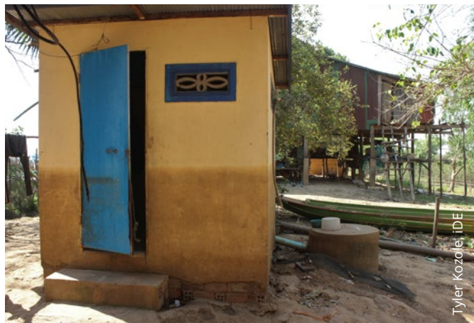
An unusual flood event in a rural village in Kampong Thom Province, Cambodia leaves a visible high-water mark on the latrine shelter. The flood water inundated the latrine pit, causing the system to overflow and become dysfunctional.
