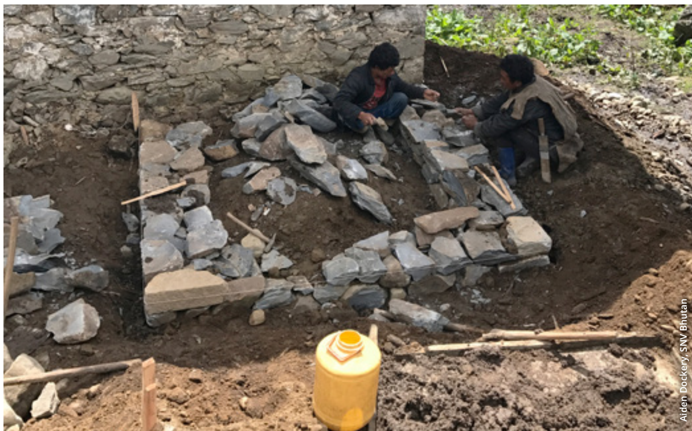
Figure 20. Toilet construction in remote mountain villages.
