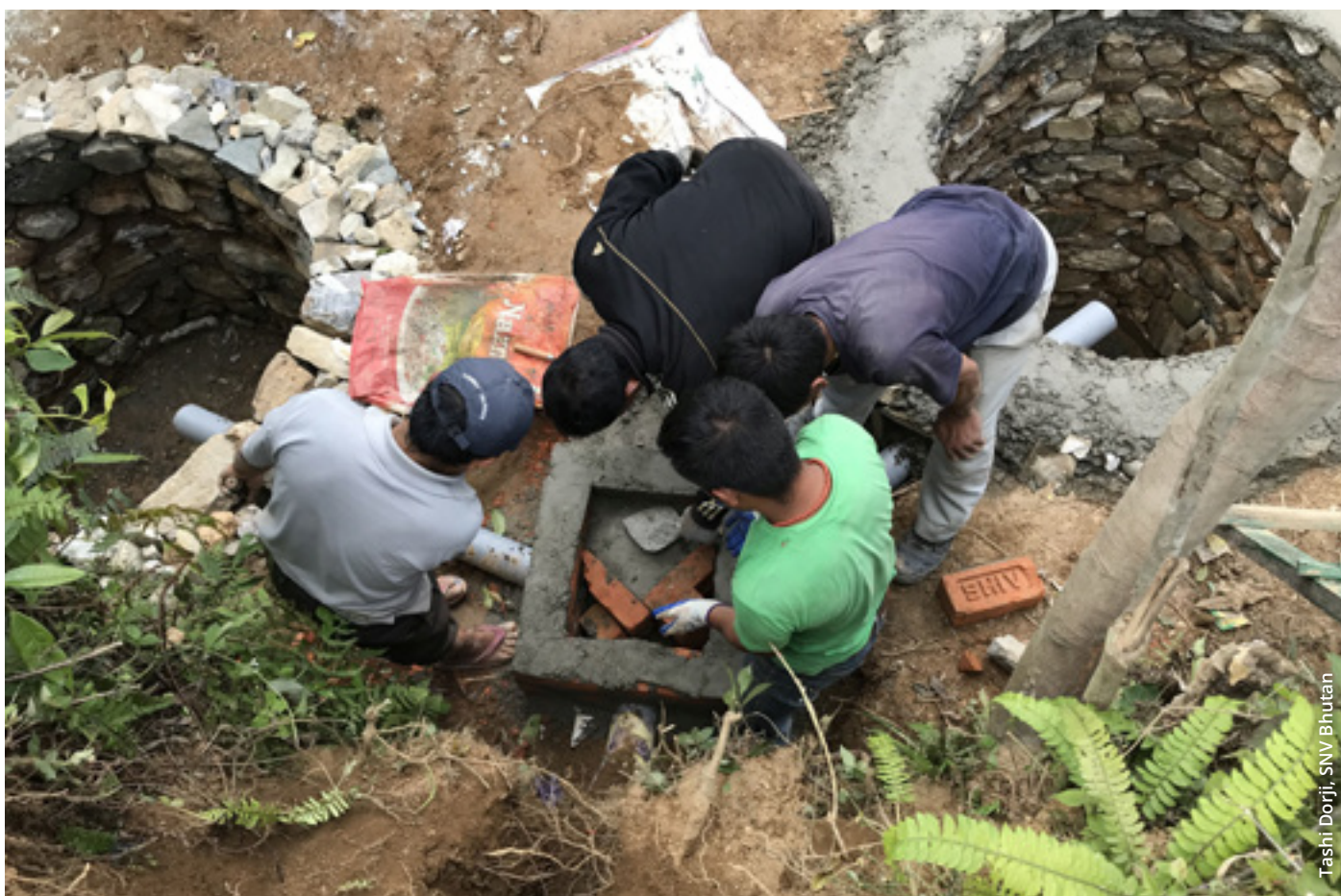
Figure 22. Installation of diversion chamber as an effective approach to safe faecal sludge management in rural communities.
