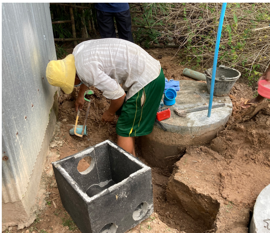
Local suppliers and masons install a twin pit latrine designed by EMW in Cambodia Credit: Thrive / EMW
