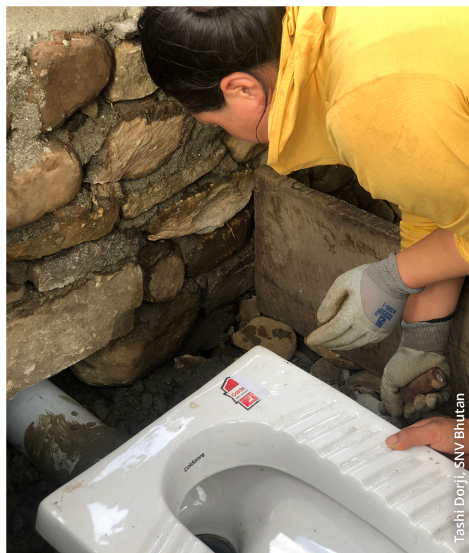
Toilet construction, Bhutan.
