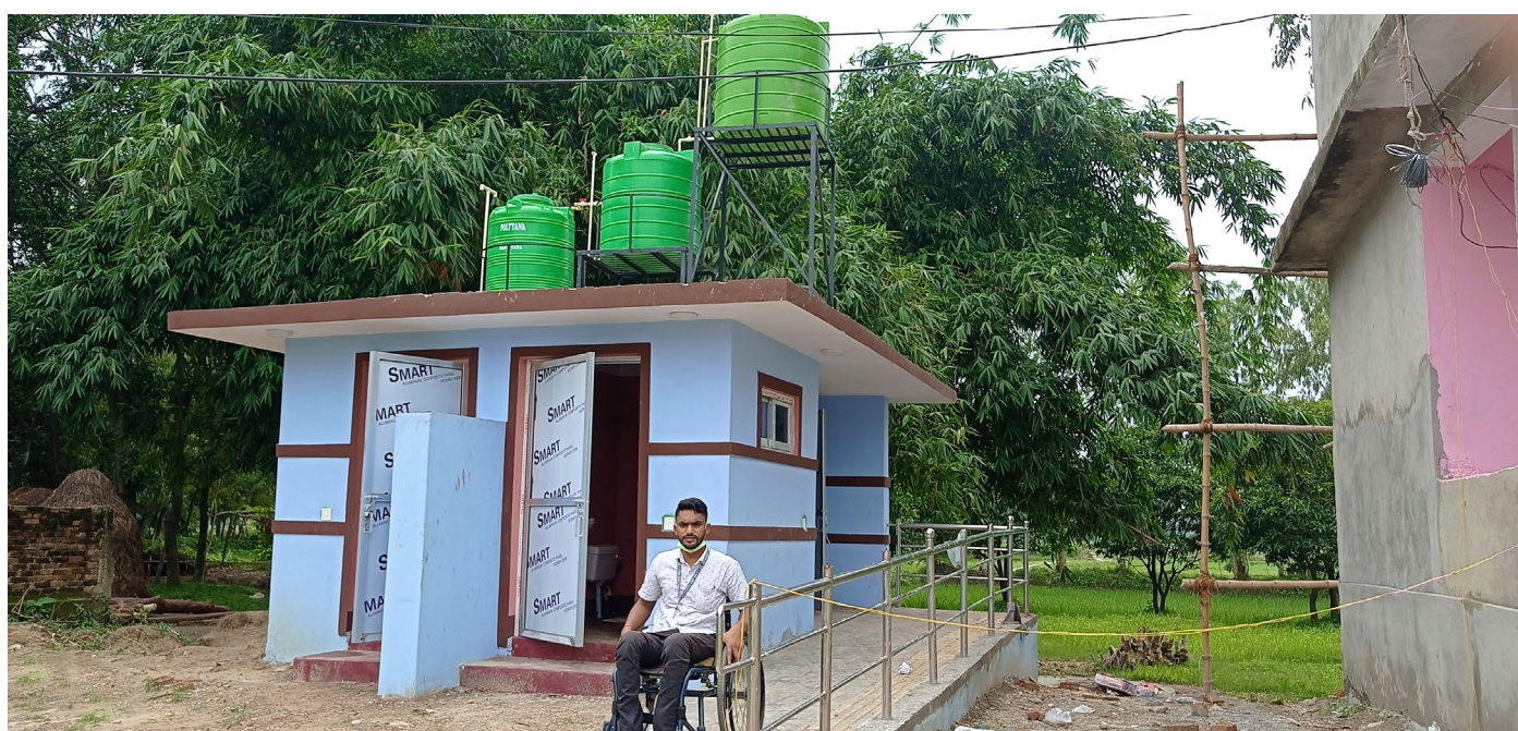
In Sarlahi, Nepal, SNV has been improving WASH outcomes by improving WASH in HCFs, including installation of inclusive latrines like this one at Parsa Health Post Credit: Sapana Rana
