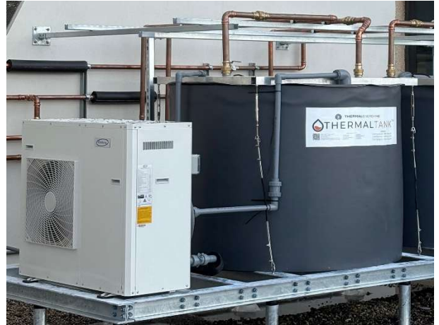
Photo: Installation site in Fort Lauderdale, FL.
