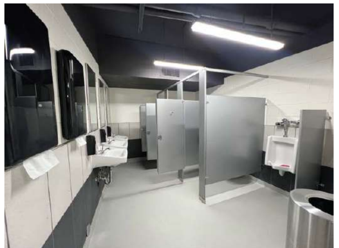
Locker Room Restrooms
