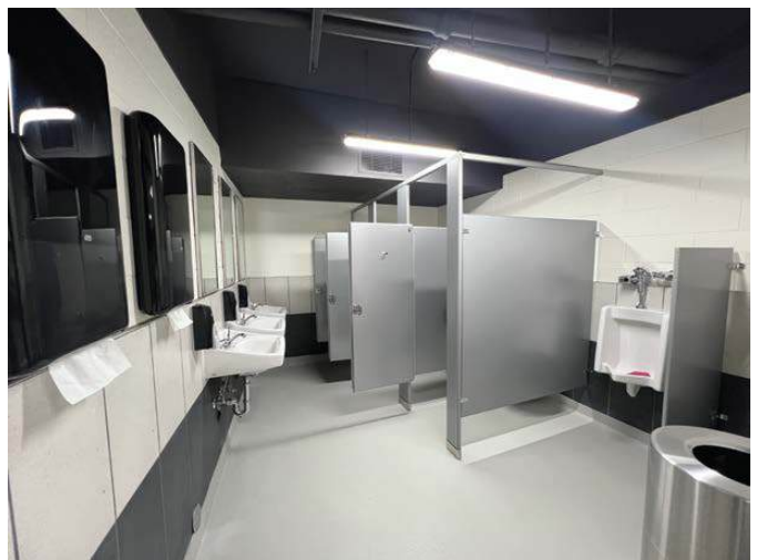
Locker Room Restrooms
