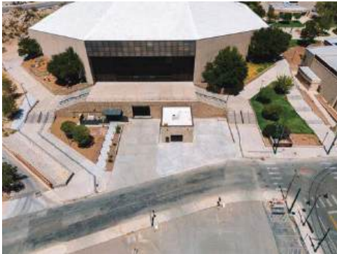
South Entrance Loading Zone Storage
