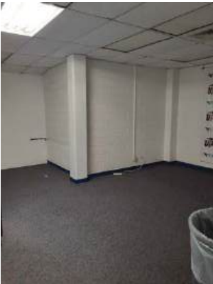
Dressing Room 3 Entrance View
