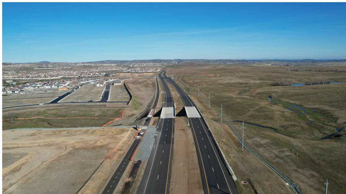
#3 - WHITE ROCK ROAD EXPRESSWAY PROJECT - PHASE 2
