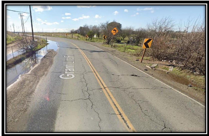
Figure 1: Current curve on the roadway facing southwest
