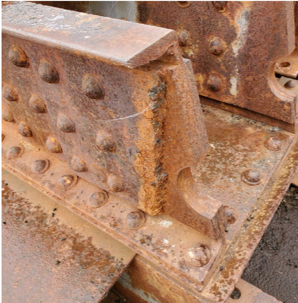
Figure 16: Cut Truss Top Compression Chord Connection Plates
