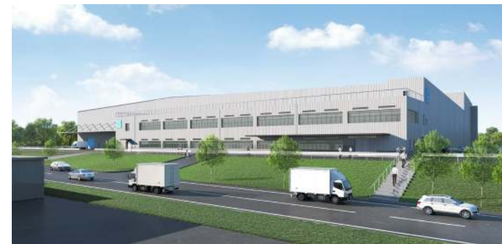
New facility within Shiga Works (rendering)
