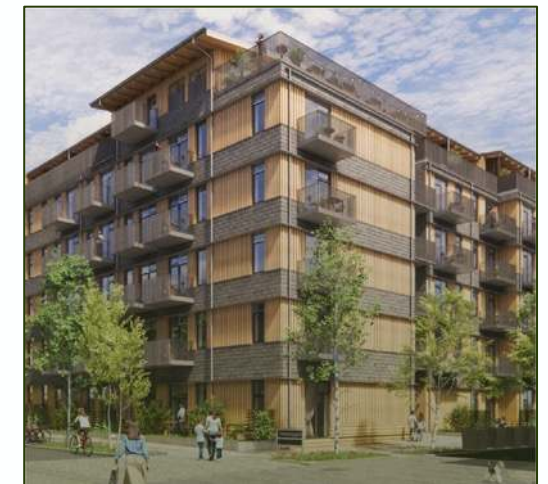
HTC, 163 homes – in construction
