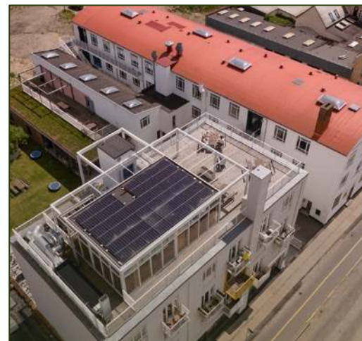
Filmlageret, 46 homes – in operation
