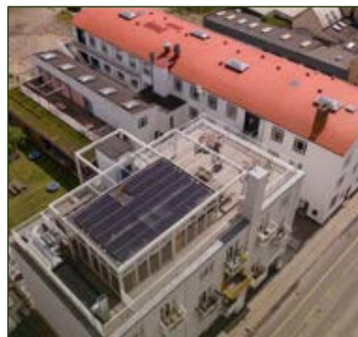
Filmlageret, 46 homes – in operation
