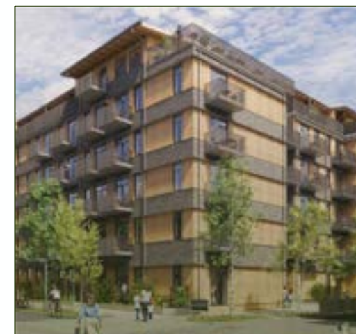
HTC, 163 homes – in construction
