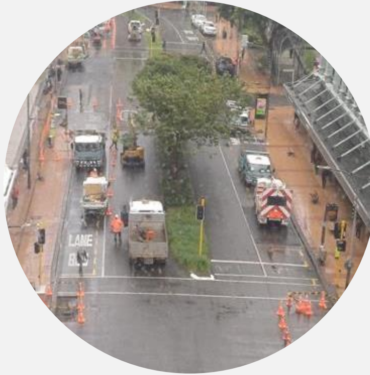
Dig outs Resurfacing Utility Maintenance
