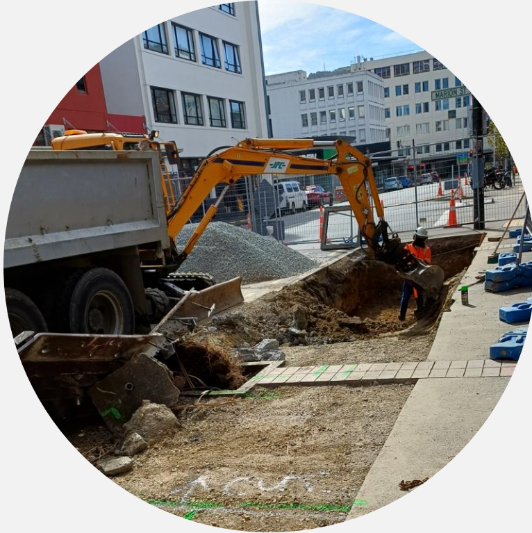
Dig outs Footpath maintenance
