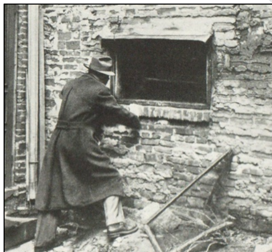
Outside view of basement Kitchen window, looking East. (Boston Public Library)
