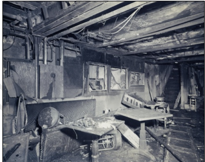
Melody Lounge, looking West toward stairs, along Piedmont Street wall. (Boston Public Library)
