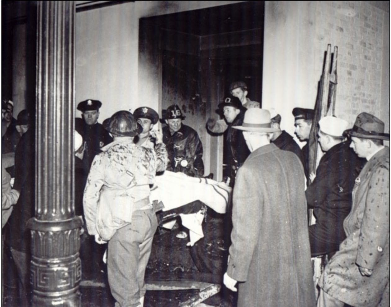
Exterior view of exit door from Lobby/Foyer, at top of stairs from Melody Lounge, looking Northwest, with Main Entrance to the right just out of picture. (Boston Public Library)
