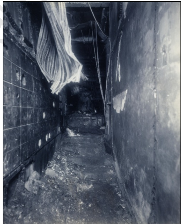
Passageway to New Broadway Lounge, looking North from Caricature bar, where fire door was required but not installed. (Boston Public Library)
